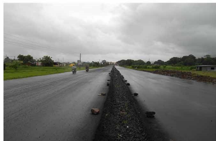
Widening of Badlapur-Karjat Road
